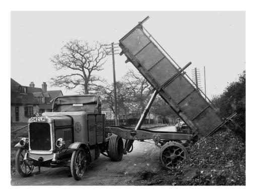
Below: The Downer tipper with large capacity trailer and coach-built cab.
