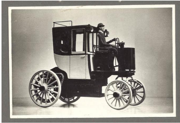
An example of a very early electric car, indicating the style of bodywork clearly taken from horse-drawn vehicles
