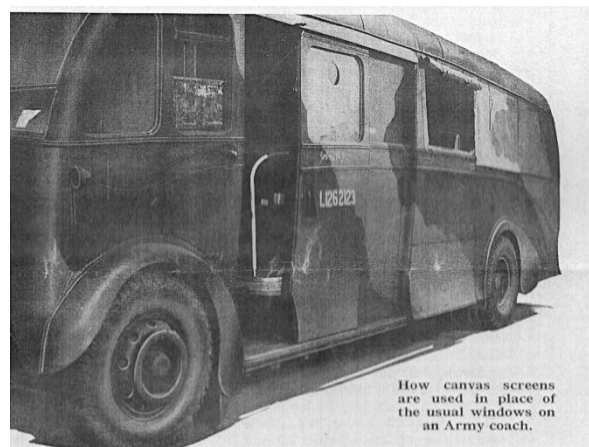
Above: A Camouflaged & 'disrupted' vehicle. Note the replacement of window glass with canvas screens (originally published in 'Bus & Coach')
