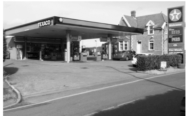
Above: 2. Frenchay Park Service Station as it was redeveloped, post-Gulf, into a Texaco self-service station with canopy. The Macs' former house is clearly seen to one side
