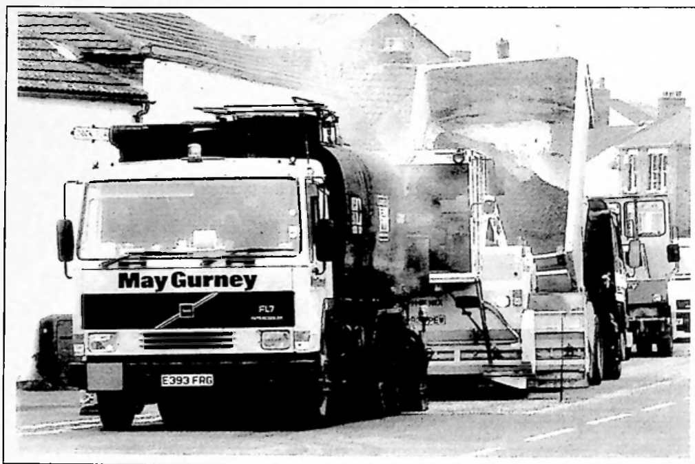
ABOVE: The way road surfacing is done today. This photograph was taken by Arthur Ingram in Chatteris in Summer 2000. The sprayer now uses a bitumen mix, the chippings are spread mechanically, and then are pushed in by the rubber tyred roller. The process is quick and causes minimum delay.
