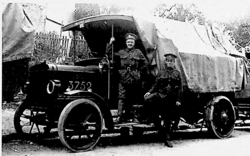
LGOC B-type 30-cwt. 3752 is the WD number and the painted out LGOC fleet number can be seen as B2511 showing it as one of the omnibuses that had the body replaced with a general service body.
