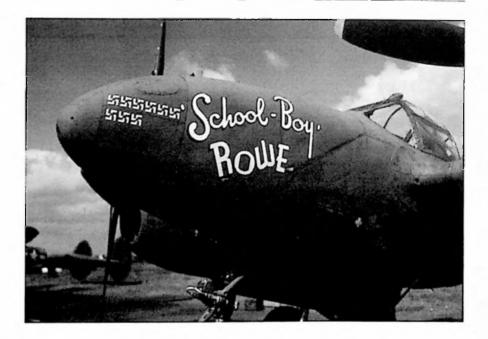
a famous baseball player at that time. It was the second plane given the name. If you look at the nose of that F-5C, you will see that the cannon mountings have been blocked off, the guns having been removed to save weight. With all unnecessary equipment removed except the camera under the nose, the plane was so fast it was almost impossible to catch. The blue paint was a special zinchromate mix which rendered the planes virtually invisible at high altitude.
