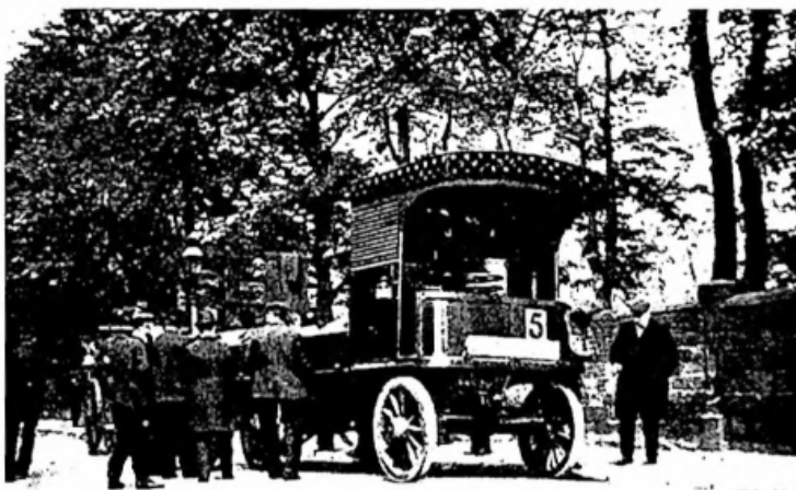
14 hp forward control Leyland 4-tonner, weighing 3.15 tons attracted much interest when entered in the 1898 Liverpool Trial.
